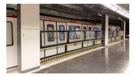
Vertical platform screen door modules in the Barcelona metro for the pilot test
